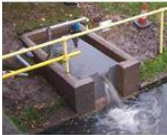
V Notch Weir
